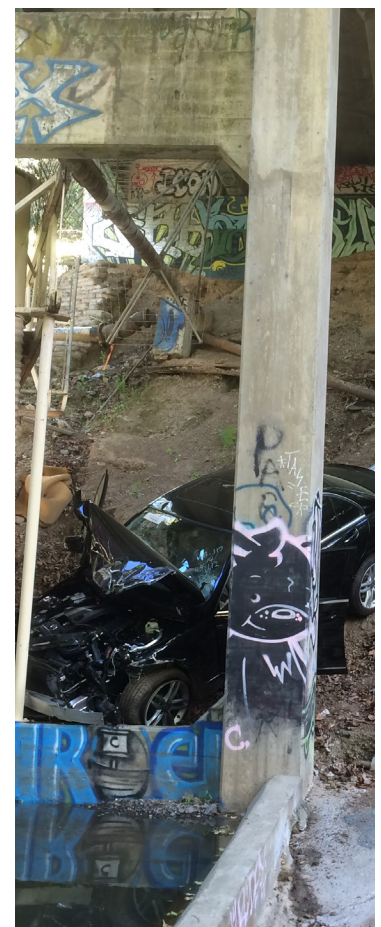
Vehicle accident at Valley Water facility.
